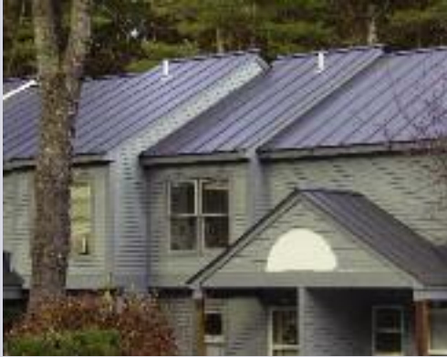
After with New Metal Roofing based on KYNAR 500® FSF®
