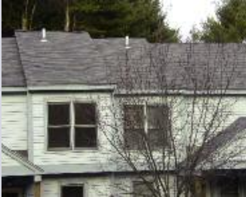
Before with Old Asphalt tile roof
